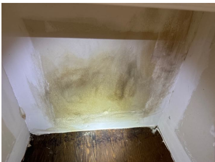
Hall closet ceiling
